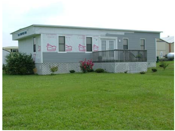
New Siding Installation – Work in Progress
